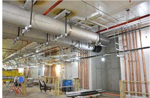
A view of cryo line installation in the tunnel.
