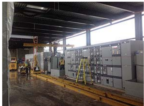
Some of the electrical substation pieces have been set.
