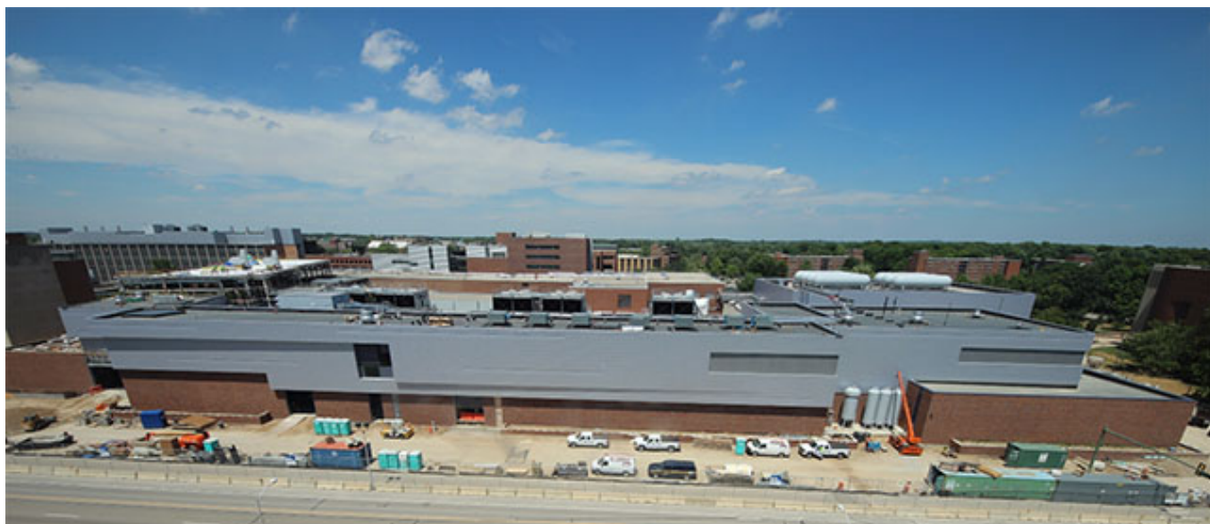
A view of the FRIB construction site on 12 July 2016.
