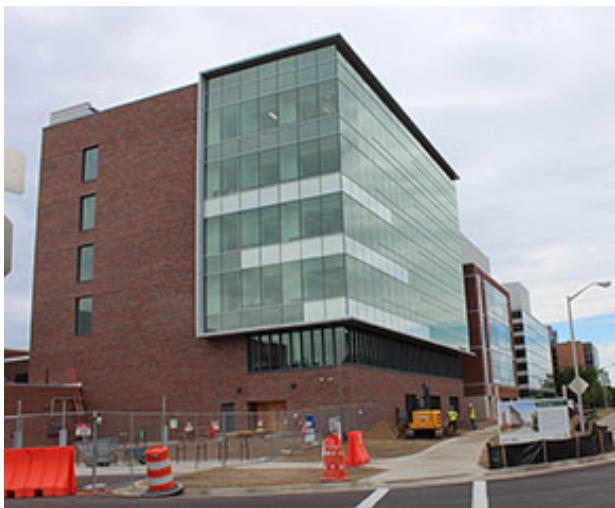
The FRIB office tower addition is advancing quickly toward August 2016 completion.
