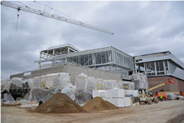
A view of the FRIB construction site. Civil construction is 10 weeks ahead of schedule.
