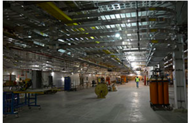
A view of the linac tunnel, one area where mechanical, electrical, and plumbing work is underway.
