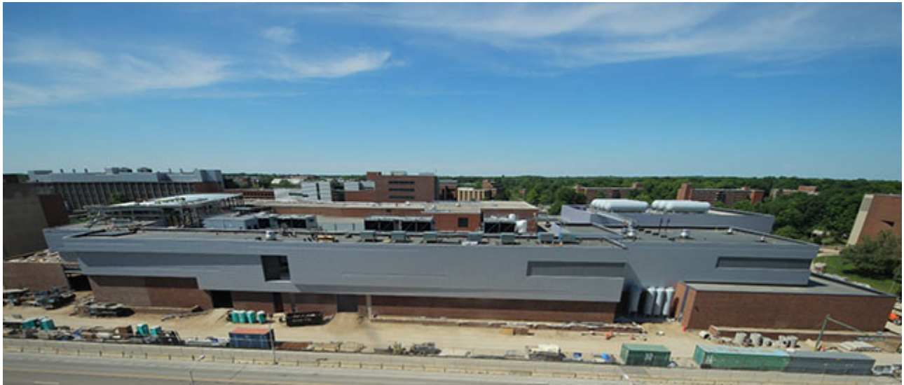
A view of the FRIB construction site on 13 June 2016.
