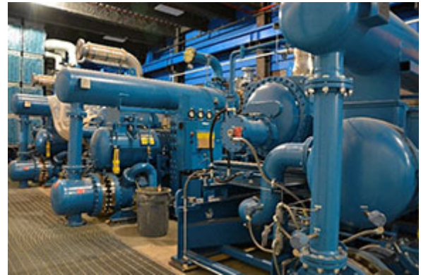
This photo shows three of six helium compressors installed in the FRIB construction site.
