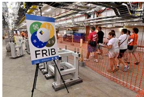
Tours were held in the currently operational experimental areas in NSCL that will be used in FRIB experiments, and visitors could tour the FRIB facility under construction.
