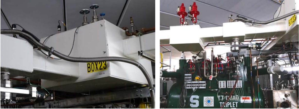
Figure 11.2 (a) NSCL Box 23 similar to proposed HRS Branch Box 2; (b) NSCL local valve box and transfer line section similar to proposed local HRS cryogenic boxes and transfer line
