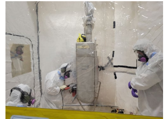
Cutting/grinding of cryomodule end-can in decontamination tent
