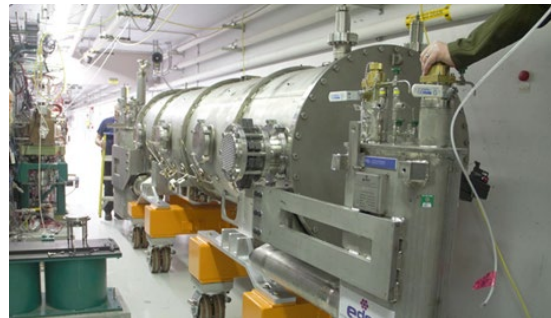
Installation of the spare medium beta cryomodule in the slot 1 in February 2020
