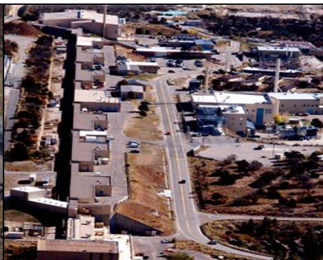
Los Alamos Neutron Science Facility (LANSCE)
